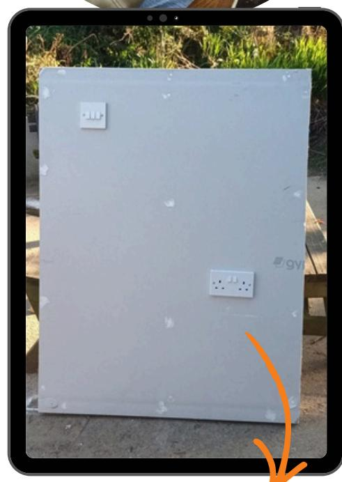
The group constructed this "Template Wall" by mounting a real light switch and double socket onto a plasterboard frame.
